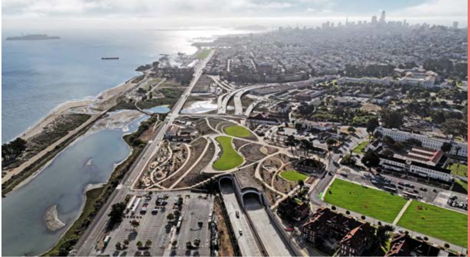
FIGURE 1: AERIAL VIEW OF THE PRESIDIO TUNNEL TOPS COVERING THE HIGHWAY 1 TUNNELS.
