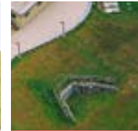
Ventilation Through Berm
