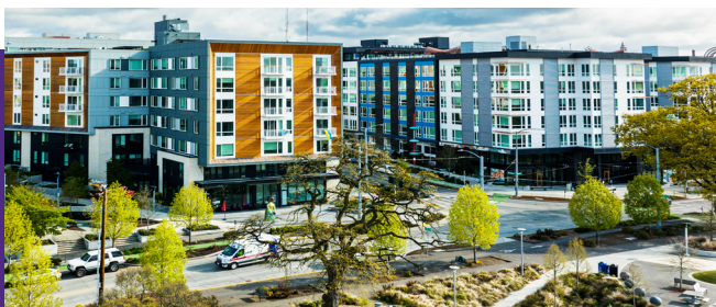
Yesler Terrace Multi-Family Housing in Seattle.
